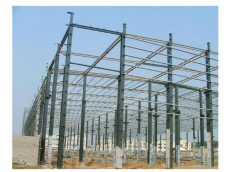
钢结构工程 Steel structure engineering
